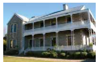
No.7 Worcester Street, Grahamstown
