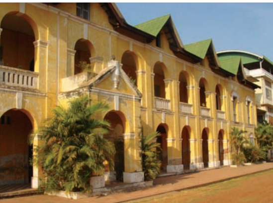
Catholic Church building, Phnom Penh
